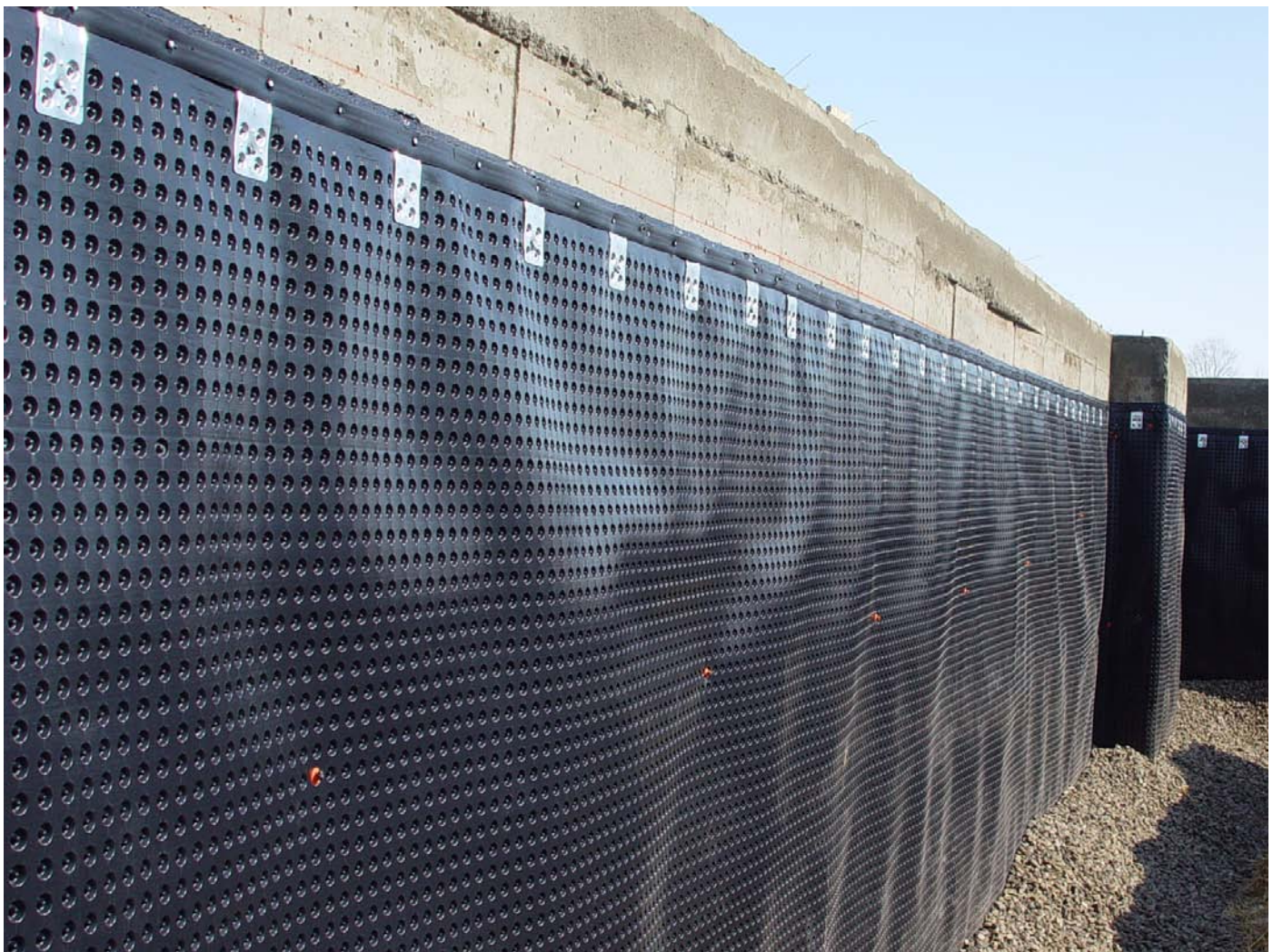
FINISHED INSTALLATION OF PLATON FOUNDATION WRAP
