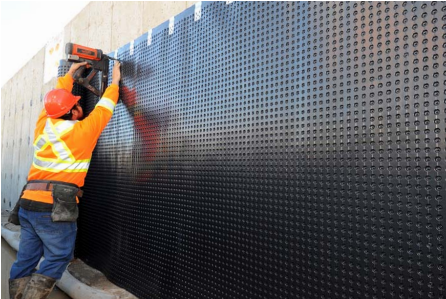
INSTALLING SPEEDCLIPS EVERY 30CM (12")
